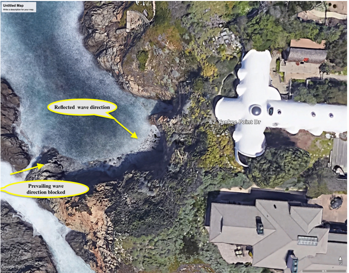
Aerial imagery (2023) showing the pattern of prevailing wind driven surf (toward the east and northeast) and large bedrock outcrops which provide a buffer between the waves and the bluff. Surf within the alcove is largely from reflection of waves off of nearby outcrops. Source: Google Earth
