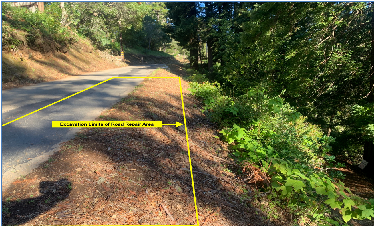
Upper section of proposed hilfiker road repair (April 23, 2026).
