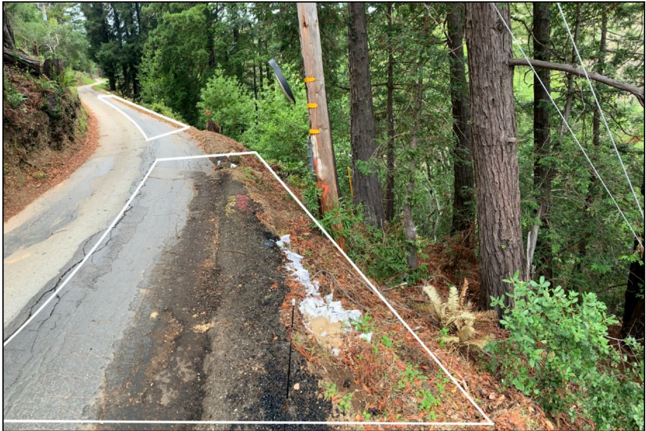
Upper (130-LF) and lower (50-LF) sections of hilfiker road repair area.
