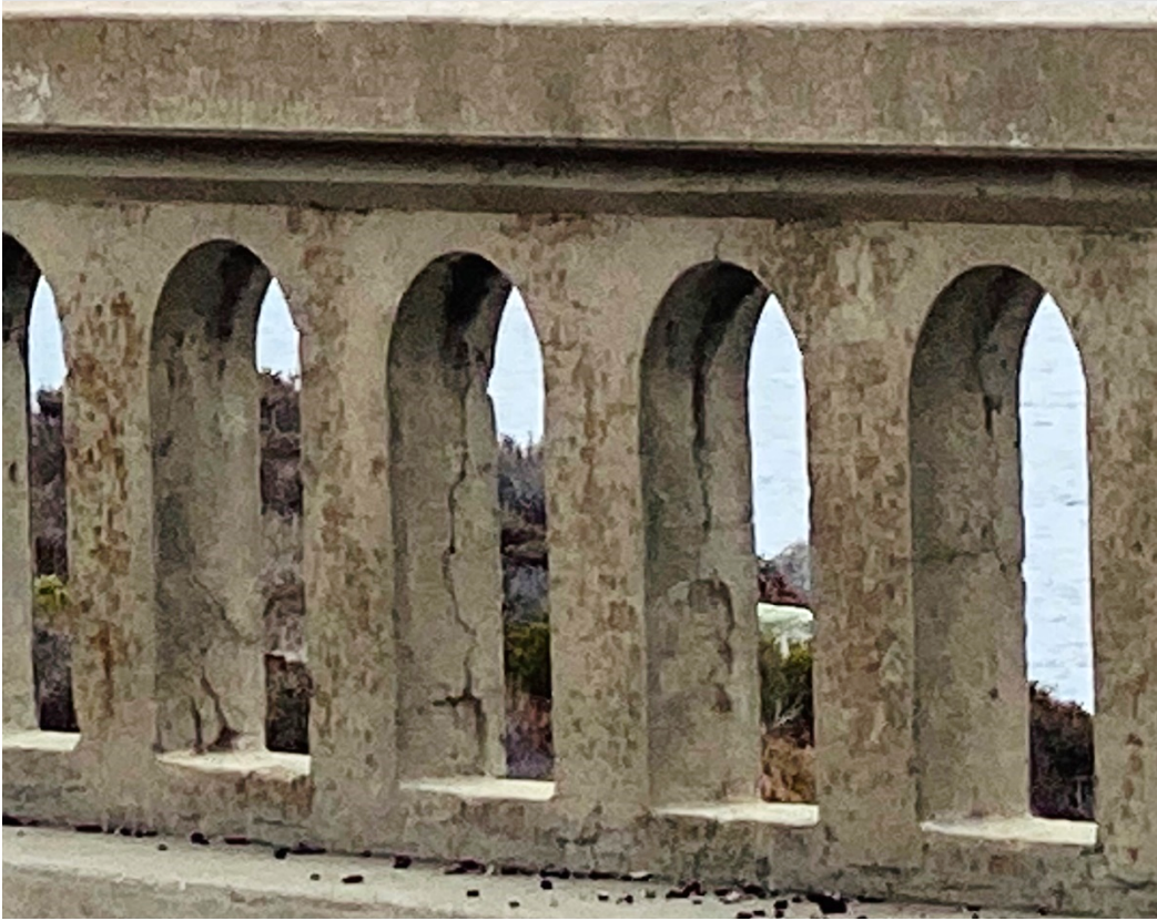
Figure 1-7 Photo of Malpaso Creek Bridge Rail Deterioration
