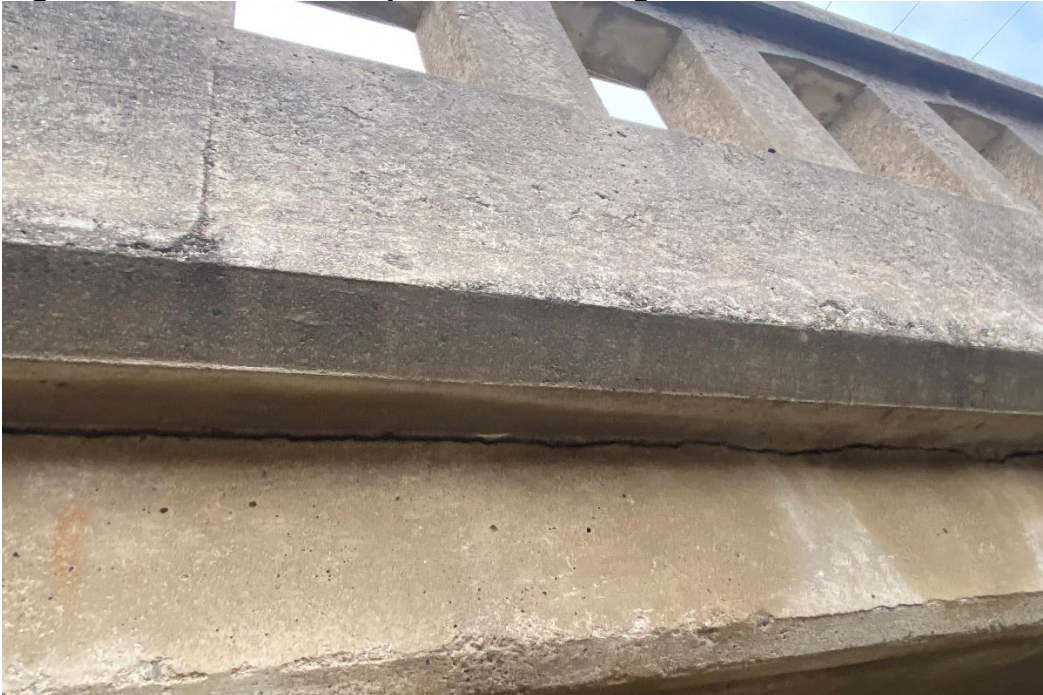
Figure 1-7 Photo of Malpaso Creek Bridge Rail Deterioration
