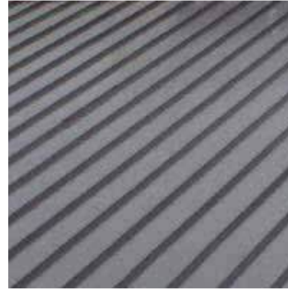
STANDING SEAM ROOFING
