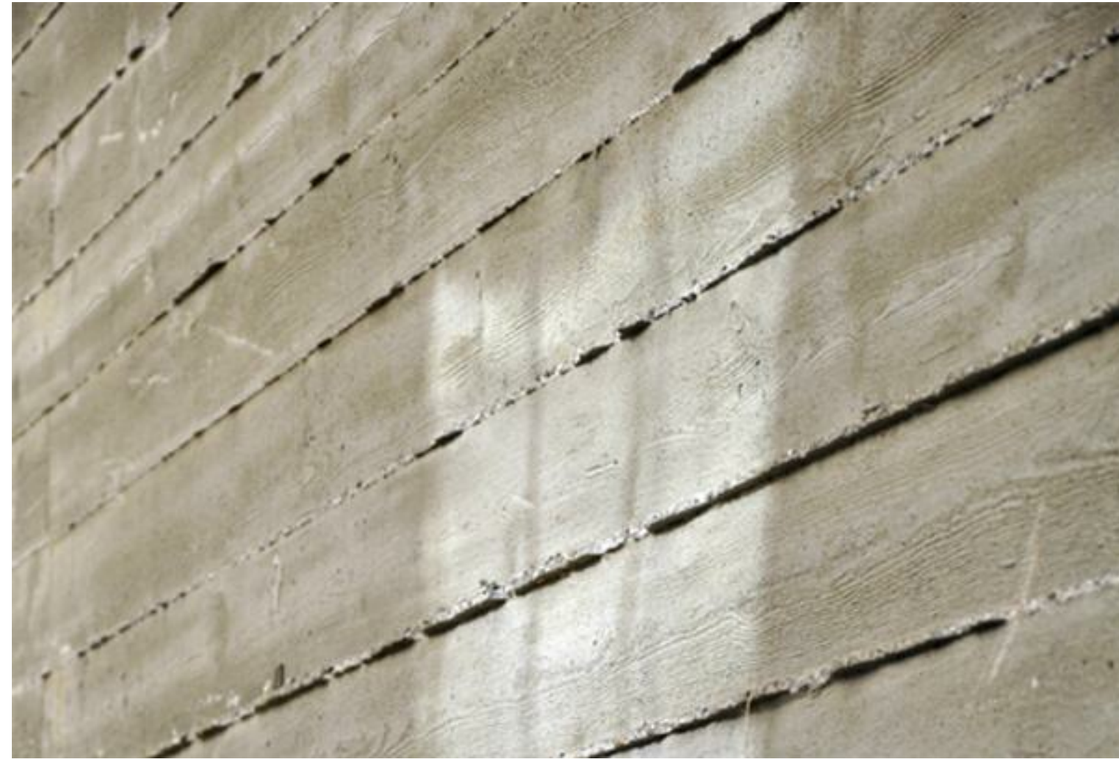
BOARD FORMED CONCRETE WALLS
