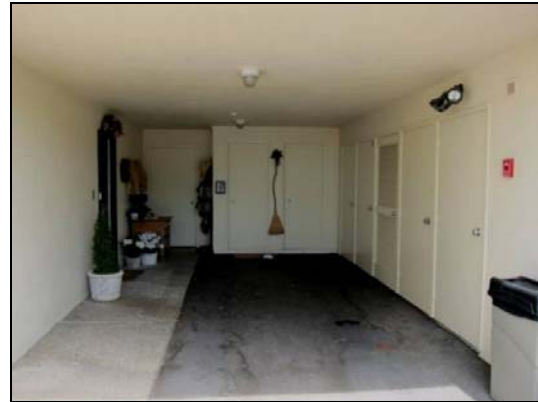
Figure 36. Typical garage design seen on Bldg. 22.
