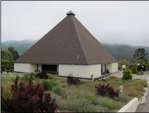
Figure 21. Side (east) elevation of Meeting House.
