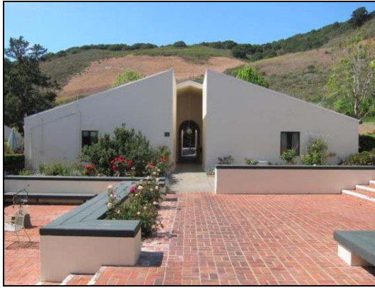
Figure 29. Front (south) elevation of the Bldg. 8.
