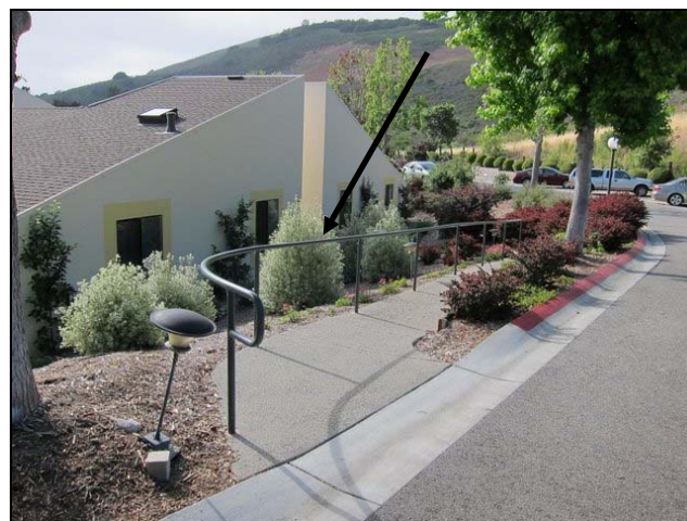
Figure 13. Example of typical railing design (arrow).
