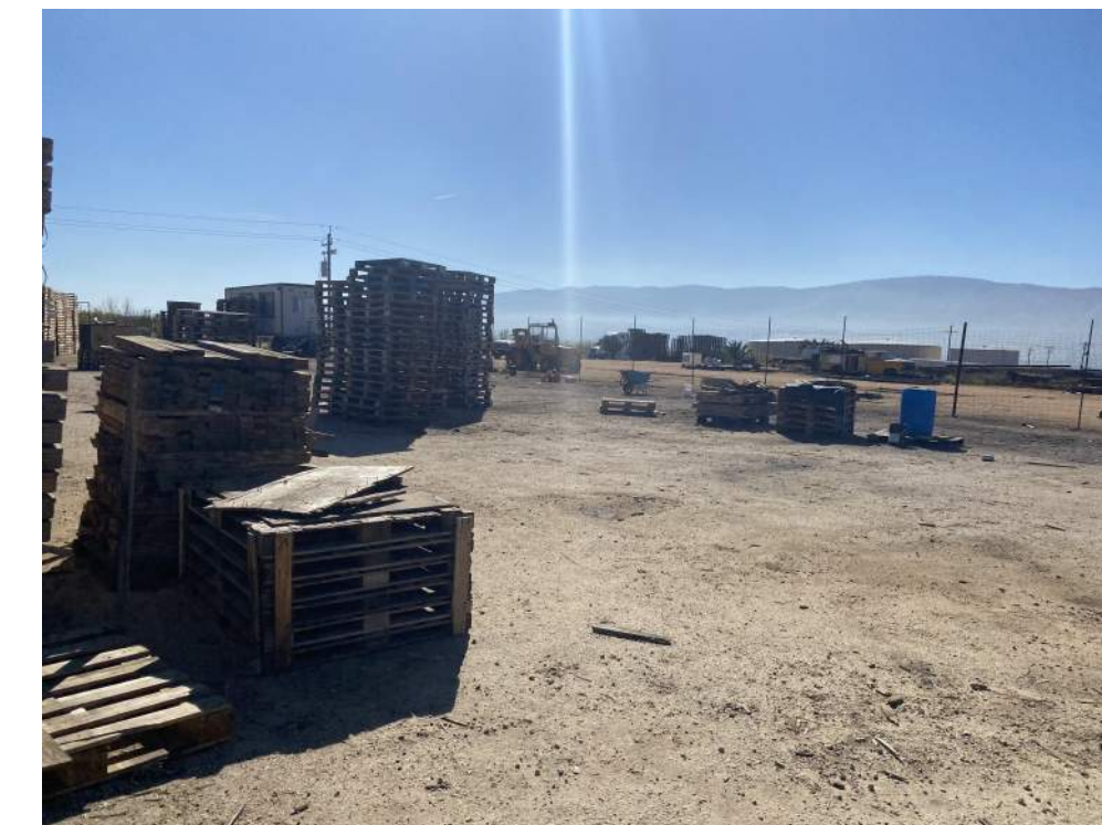
CURRENT CONDITIONS ON SITE
