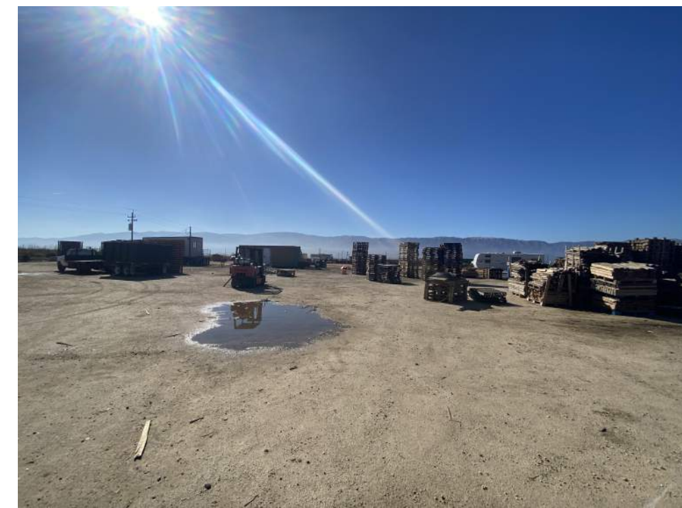
CURRENT CONDITIONS ON SITE
