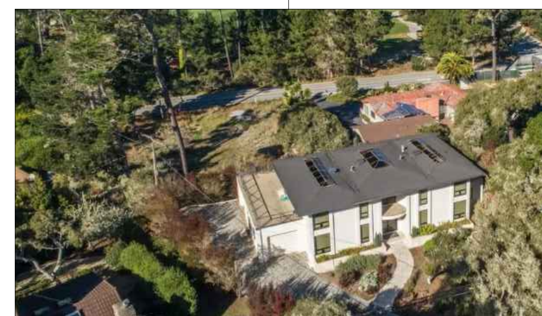
2900 OAK KNOLL ROAD - AERIAL VIEW
