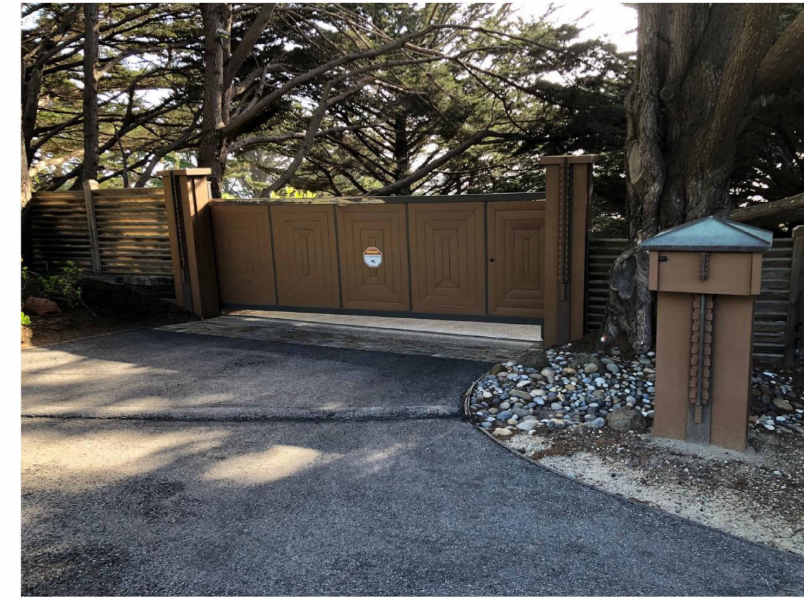
MAIN ENTRY GATE
