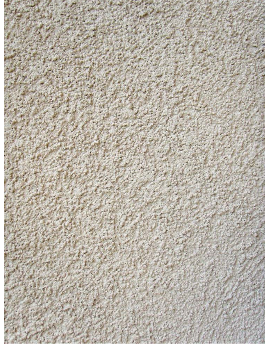
EXTERIOR SITE WALLS: STUCCO OVER CONCRETE
